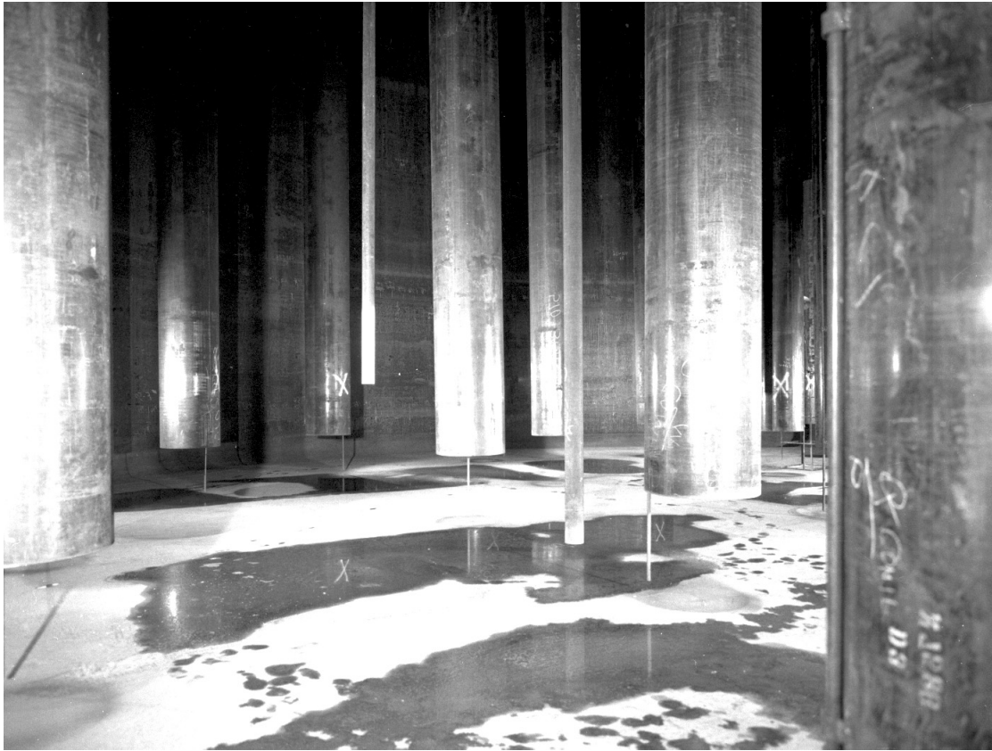
Figure E-3. AX Farm Tank During Construction
